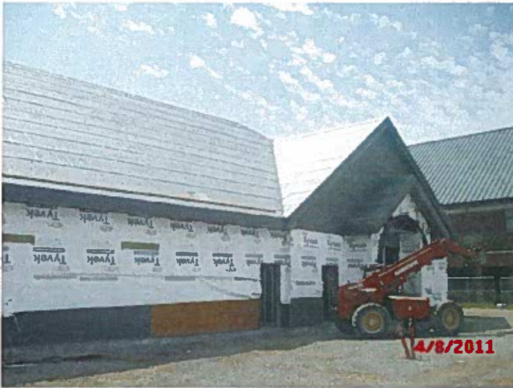
CSC Student Center - NW corner of the building.
