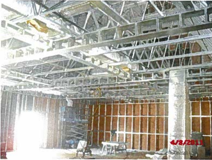
CSC Student Center - Soffits and Duct above the library.
