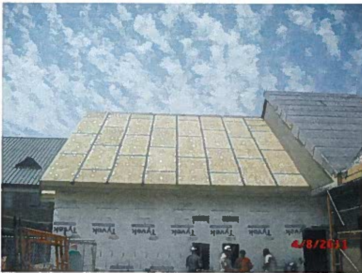
CSC Student Center - South end of the office area.
